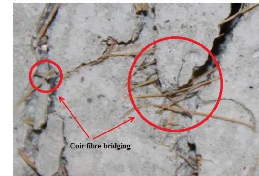
Coir fibre bridging: reduce concrete cracks & modify failure concrete to be ductile
